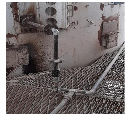
2nd feeding point of low NCV feeding point at oxidising zone
